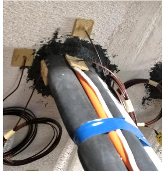
Mixed services treated with FYREPEX™ Sealant in a Hebel wall
