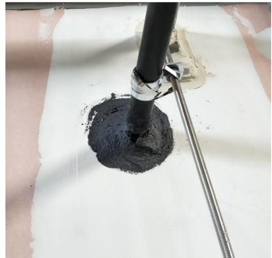
PEX pipe treated with FYREPEX™ Sealant in a Plasterboard Wall
