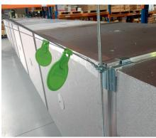
**Gripple seismic bracing systems** are used to restraint most non-structural components. When used in conjunction with the ALP system it is possible to greatly reduce the size of the braces due to the lightweight nature of this component.
