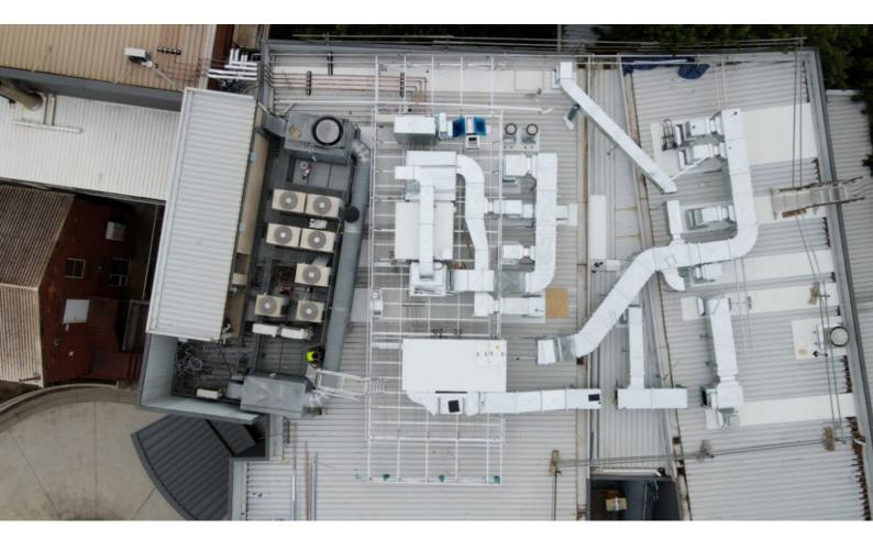
There are multiple factors we consider when engineering one of our HVAC mounting and roof access solutions. At Con-form Group, we have two types HVACR mounting systems which distribute loads in two completely different ways.
